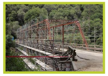
The bridge was completely enveloped in scaffolding so the Contractor could repair damaged structural bridge members. The bridge was then wrapped in a PVC tarp to protect the river and environment during the bridge painting process
